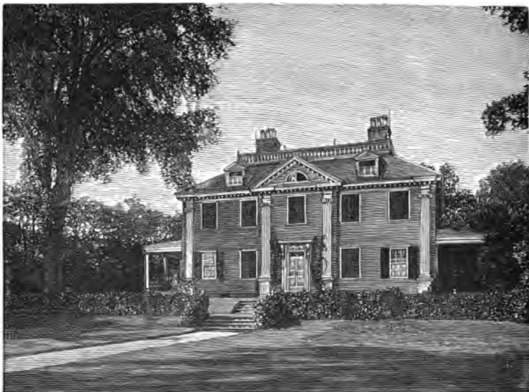
THE CRAIGIE HOUSE, WASHINGTON'S HEADQUARTERS AT CAMBRIDGE (AFTERWARD THE RESIDENCE OF LONGFELLOW).
